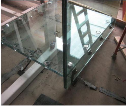
Figure 9: Mock up of Wall and Floor Panel
